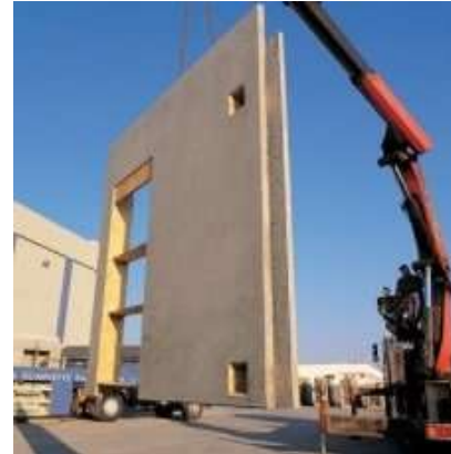
F. 14.1.3.1 Precast Flat Panel System
