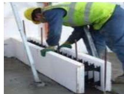
F.14.1.3.6 Insulating Concrete Formwork
