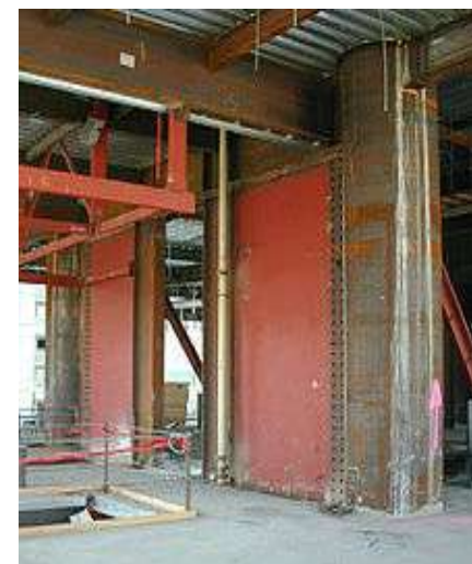
F.14.1.1.3 Steel Plate Wall System
