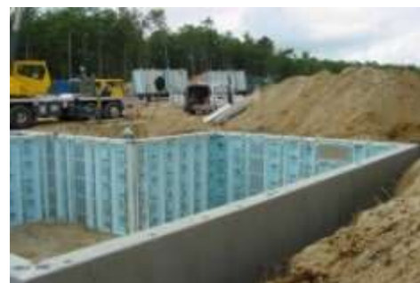
F. 14.1.3.3 Precast Concrete Foundations
